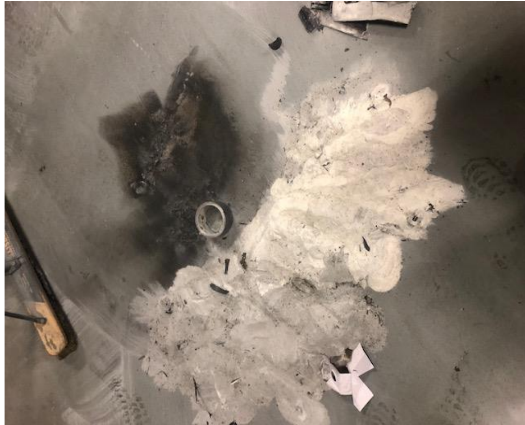
Facility floor in Storage area
