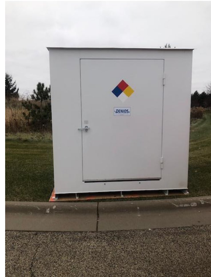
New Storage area
